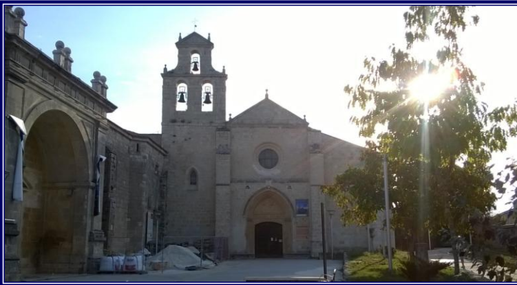
Basilica of San Juan de Ortega Restoration in progress
