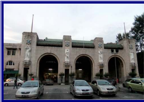
The Railway station at Tanjong Pagar.
