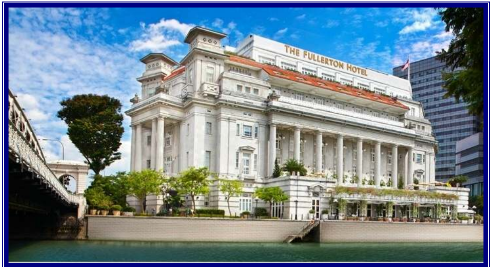
2011 What a difference 47 years make! The Post Office, reinvented as the Fullerton Hotel, with Anderson Bridge to the left of picture
