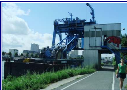
A coal barge unloading for the EDF power station
