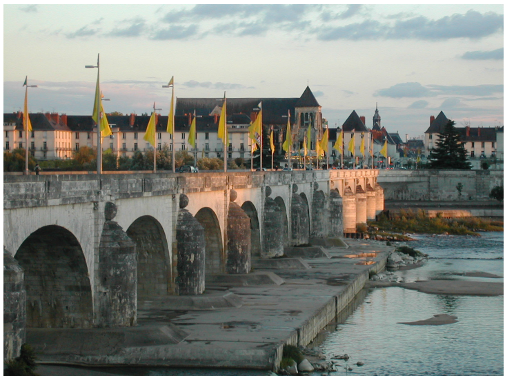
Bridge over the Loire at Tours
