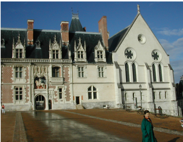
Figure 13 - Blois, East façade
