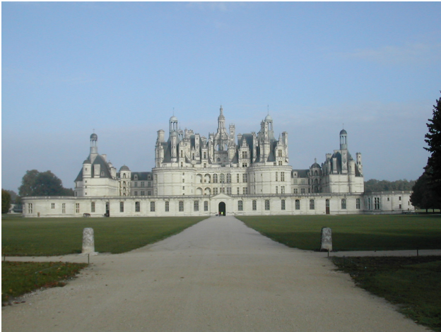
Figure 11 - Chambord, North Façade
