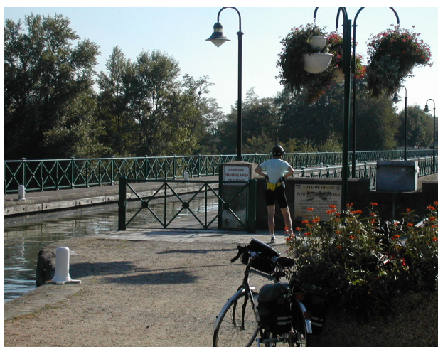
Figure 7 - The Pont-canal at Digoïn
